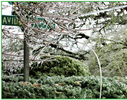
Downed primary electric line
